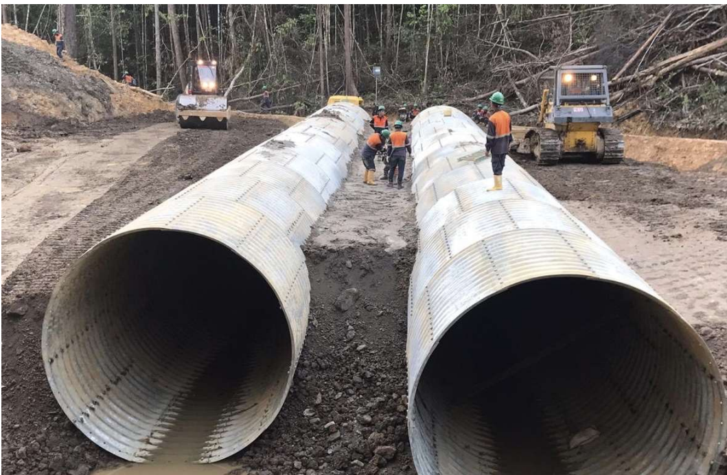
Water management culverts being installed for new haul roads.
