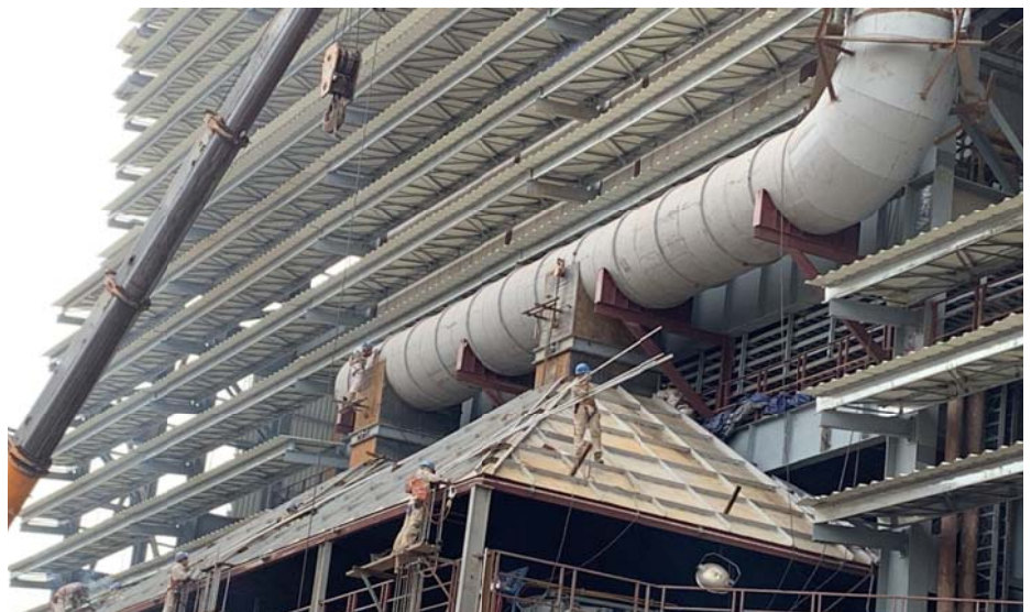
The Hengjaya Nickel Project under construction within the IMIP
