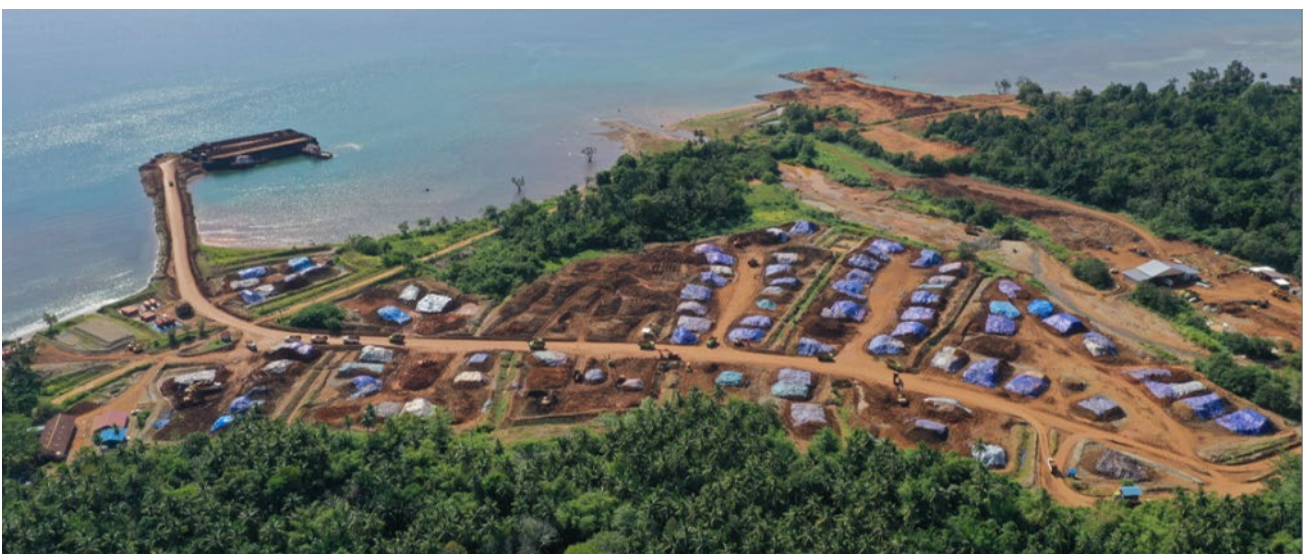
Stockpiles and jetty operating at 2.5 mtpa
