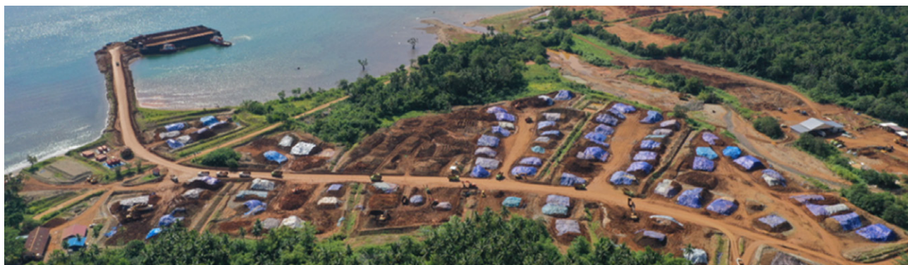
Stockpiles and jetty operating at 2.5m tpa
