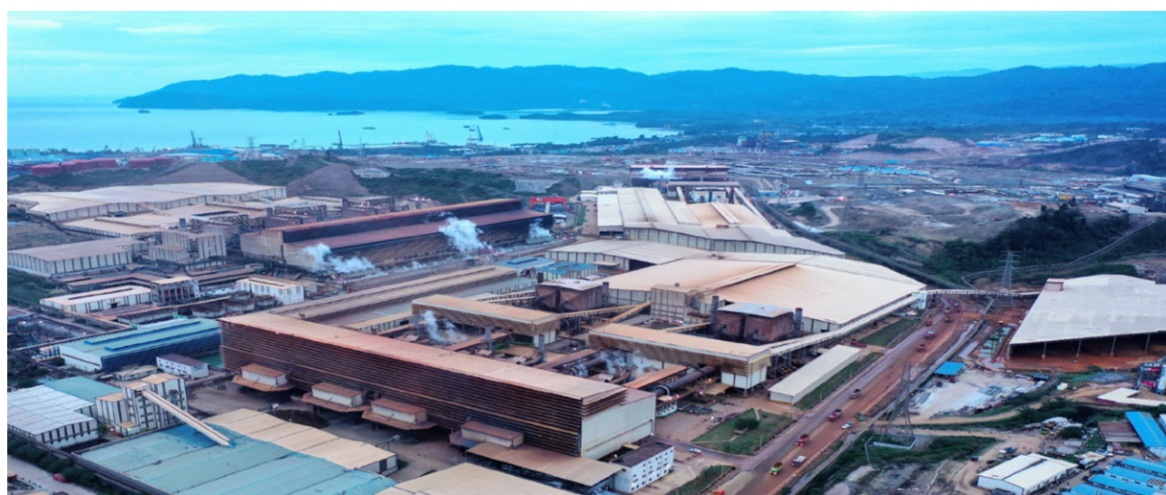
Hengjaya and Ranger RKEF operations
