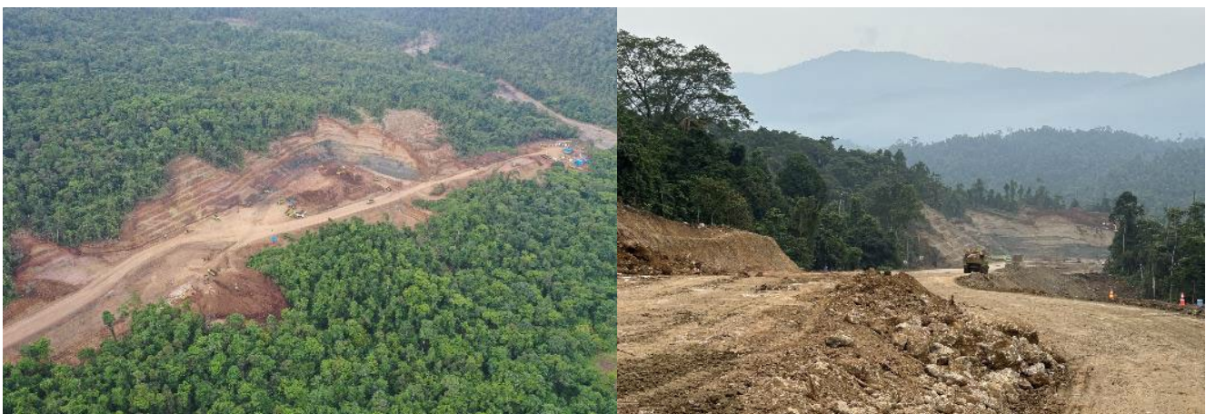
APL segments of haul road to IMIP under construction
