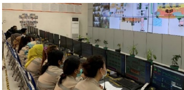
Control room at Angel Nickel
