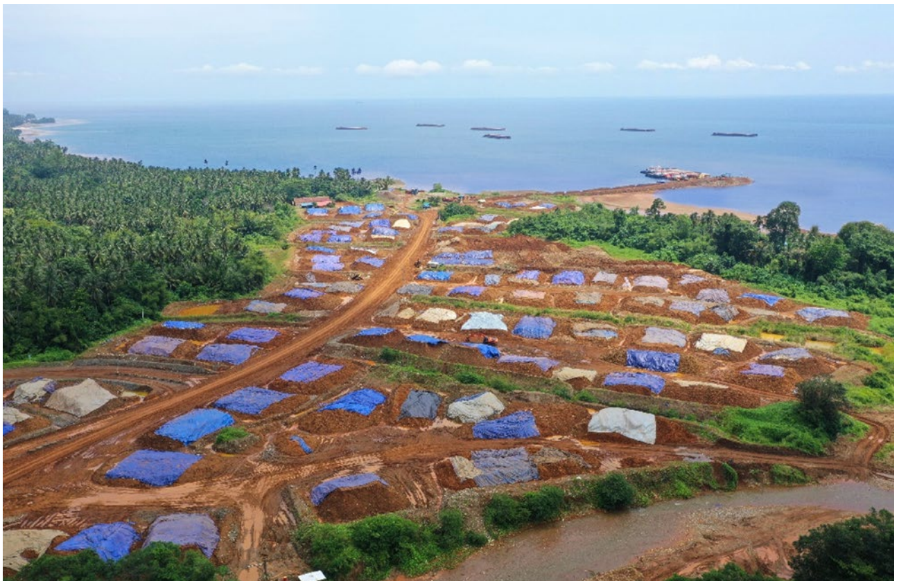
Stockpiles and jetty operating at 3.5m tonnes per annum
