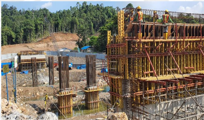
Haul road progress
