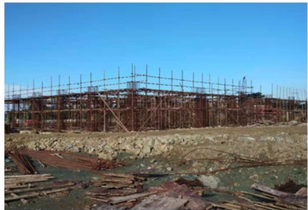
Column reinforcement for Electrostatic Precipitator
