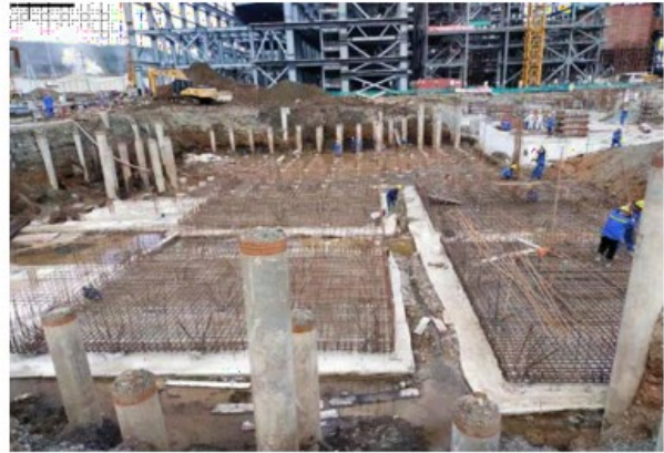
Foundations for ANI powerplant
