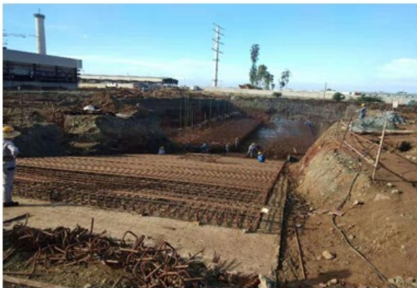
Foundations for Dry Ore shed
