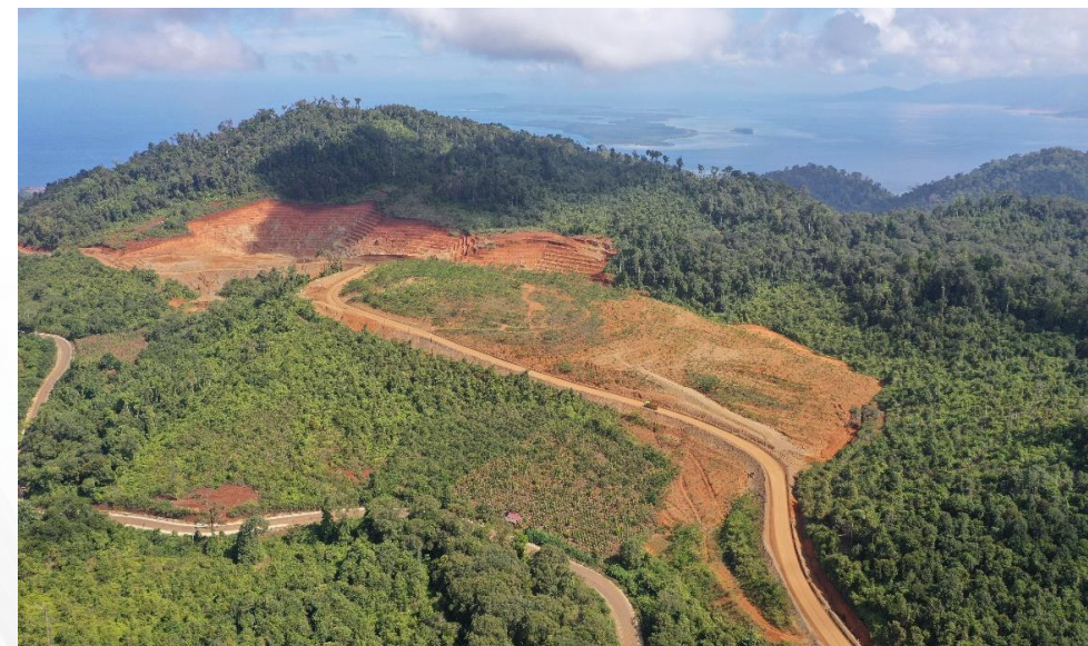
Aerial view of Central Pit 1
