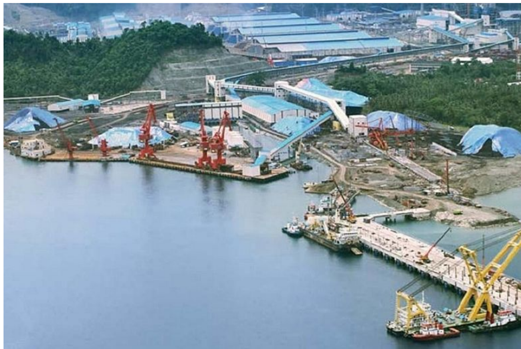
A cargo terminal in the Indonesia Morowali Industrial Park. It has its own seaport and power plants, with an airport to be completed this year. The park is expected to soon produce three million tonnes of stainless steel slabs a year. PHOTO: IMIP
